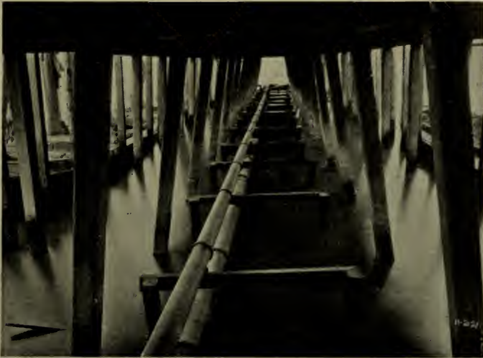
FIG. 6B. WOULDHAM CEMENT CO.'S UNLOADING JETTY: VIEW UNDER DECK.
